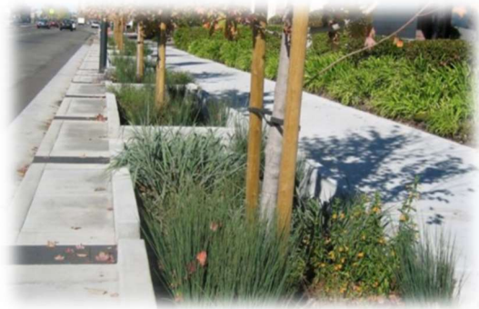
Figure 2.10. Bioretention planters in El Cerrito, United States (source: http://www.madrono.org ).
