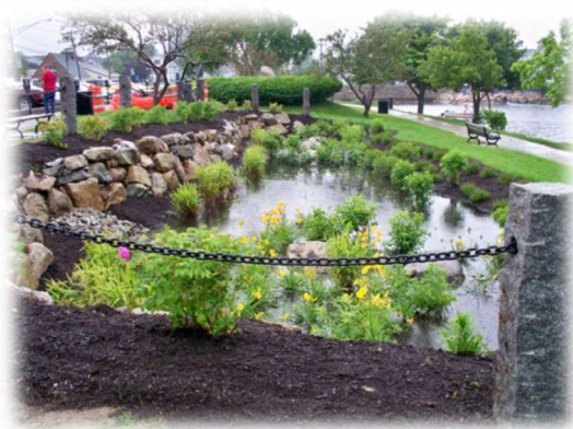
Figure 2.8. Bioretention basin at Water Street in Plymouth Center, Massachusetts (source: http://capecodgreenguide.wordpress.com ).
