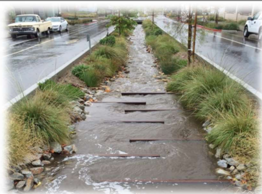
Figure 2.9. Infiltration trench in Paso Robles, United States (source: http://www.svrdesign.com ).
